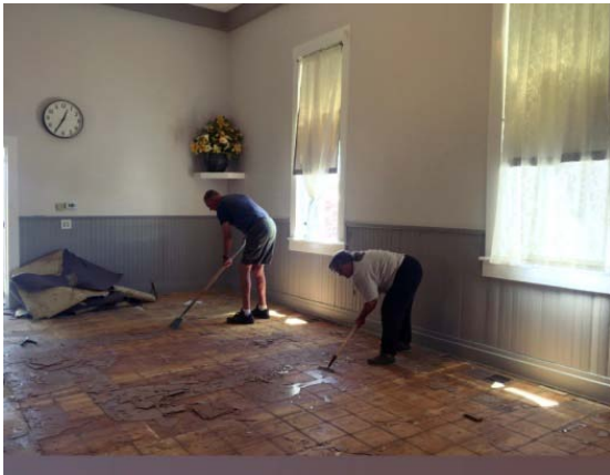
Preparing the floor by removing the old carpet and scraping away the glue.
