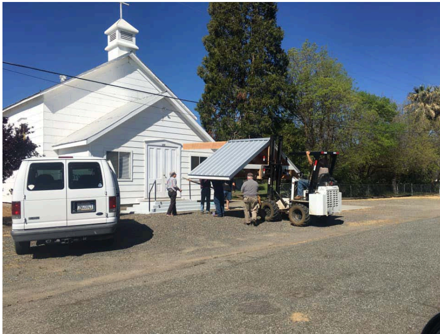
Frank Pendell, on forklift, prepares to insert the ridge pole on the overhang into the prepared cutout on the church vestibule.
