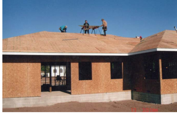
Installing the sheathing. Finished October 11, 2008
