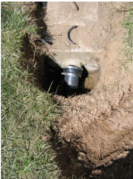
Church Septic Tank Connection.
