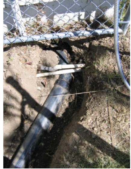
David Isle dug to reveal septic inlet leak.
