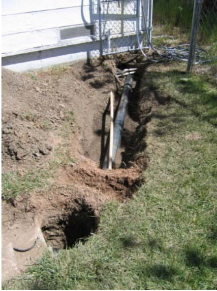
Church septic inlet leak excavation.
