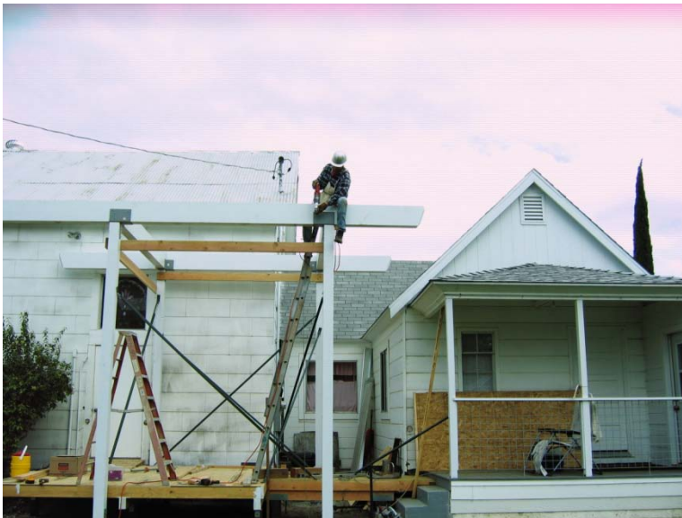
David Isle works from on high to secure the beams in place.
